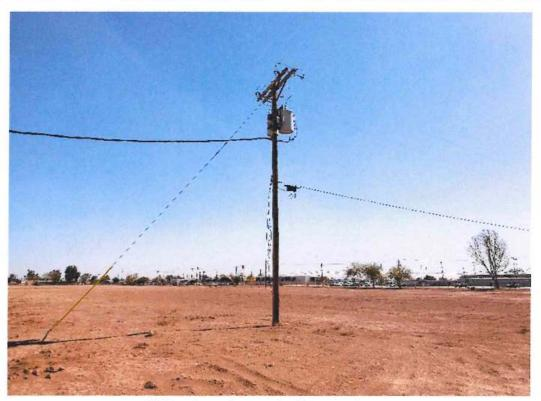
1) View of a wood power pole with two transformers.
